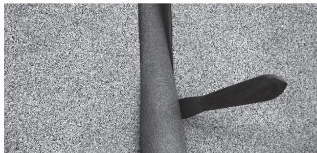
FIGURE 7.2 – INSERTING BACKER ROD
