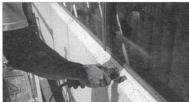
FIGURE 6.3 – POWER OSCILLATING BLADE CUTTER
