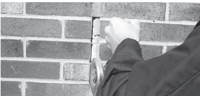
FIGURE 6.1- USING A PORTABLE GRINDER
